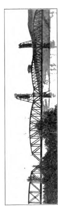
Fig. 31r. Great Northern Railway Bridge over the Yellowstone River, Montana.-Lifting Span Down.
