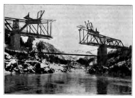
Fig. 25c. Simple-truss Bridge on the Nippon Railway in Japan, Erected by the Cantilever Method.
