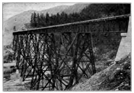
Fig. 23a. Single-track-railway Trestle over Stoyoma Creek near North Bend, B. C., on the Line of the Canadian Northern Pacific.
