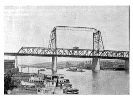
31n. Bridge over the City Waterway at Tacoma, Wash.—Lifting Span Down.
