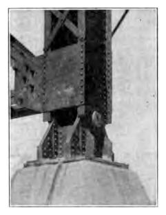
Fig. 23d. Built Rocker-shoe for a Solitary Bent in the South Approach of the Fratt Bridge over the Missouri River at Kansas City, Mo.
