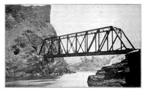
Fig. 25h. Simple-truss Bridge over the Thompson River on the Line of the Canadian Northern Pacific Railway in British Columbia, Erected by the Cantilever Method.
