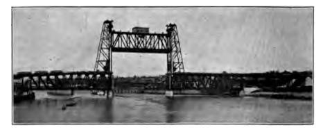
Fig. 31l. O.-W. R. R. and N. Co.'s Bridge over the Willamette River at Portland, Ore.—Lifting Deck and Lifting Span Up.
