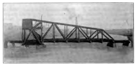
Fig. 30b. Scherzer Bascule Bridge.
