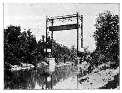
Fig. 31i. Vertical Lift Bridge over the Big Choctaw Bayou, Louisiana, on the Line of the M. L. and T. R. & S. S. Co.—Span Up.
