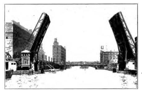
Fig. 301. Chicago City Type Bascule Bridge.
