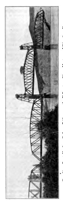
Fig. 31s. Great Northern Railway Bridge over the Yellowstone River, Montana.-Lifting Span Up.
