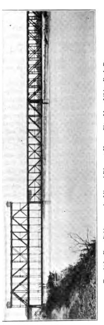
Fig. 31d. Frutt Bridge over the Missouri River at Kansus City, Mo.—Lifting Deck Down.
